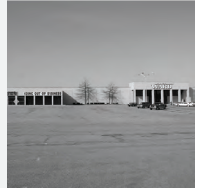
A failed shopping center:
